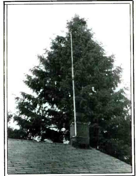
Figure 2: Austin Custom Antenna 2M/1.25M/70CM fixed tri-bander atop 8-foot PVC pipe 1" ID. Also receives well on adjacent commercial bands.
